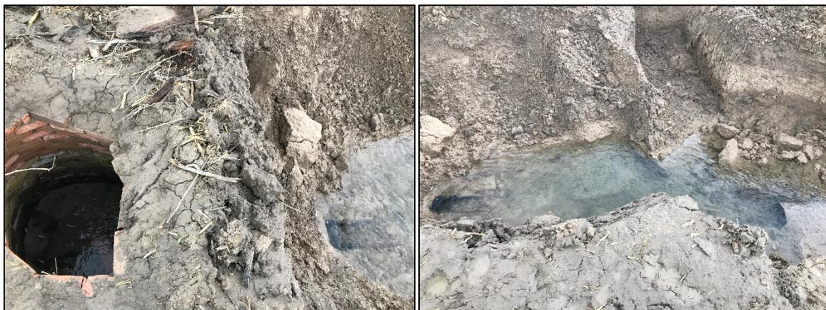
Fig 3. Photo of a manhole at the southeast section of field F1 (left panel) and the adjoining tile drain that collapsed (right panel).
