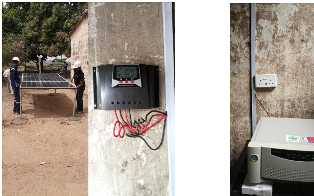
Figure 1 - Installation in Oyo State, Nigeria.
