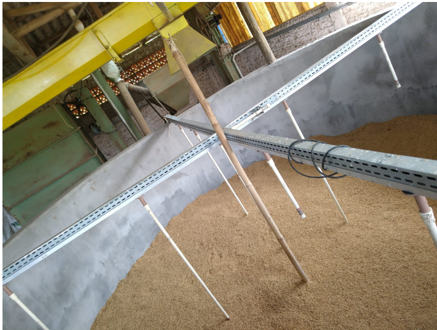
Fig 6. Sensor installation inside the silo.
