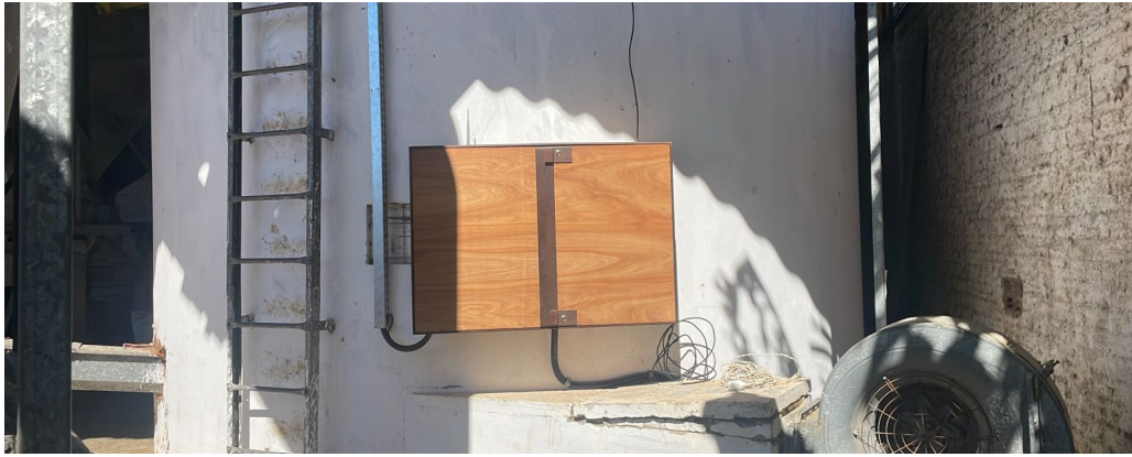
Fig 4. Small brickwork silo where the MACS was installed.
